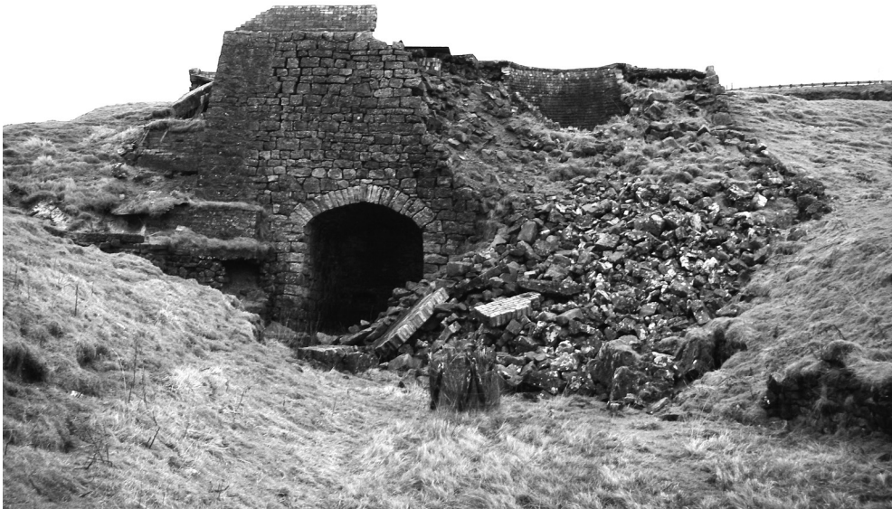
FIG. 3. semi-ruinous kiln, with segmental arch, at Well Head, North Stainmore.
