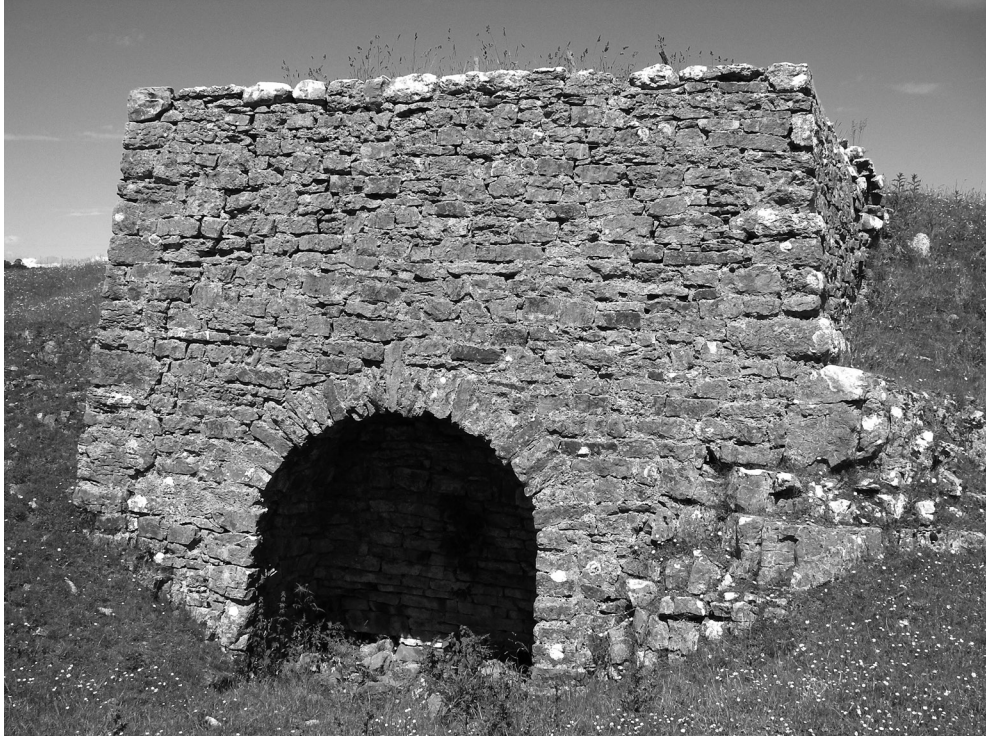
FIG. 2. 'complete' kiln, with Romanesque arch at Great Asby.
